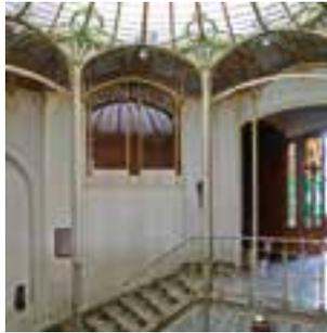
Leopold II. When building it, Horta made extensive use of exposed metal structures, an approach previously only seen in industrial construction, devising an oriel that filled the entire width of the façade over two levels. A second wing, this time in white stone, was added between 1899 and 1900. Mosaics criss-crossed by trailing creepers welcome visitors into the hallway and beckon them towards the rotunda
