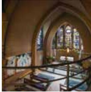
on building a new complex based on plans by architect L. Denekens. One of the new structure's wings housed a chapel, which was completed and consecrated in 1961. The chapel, made of exposed yellow brick, is formed of a single nave topped with a vaulted ceiling featuring pointed arches and soaring to a height of around three storeys. It is notable for its collection of shimmering translucent-concrete windows, which bathe its interior in warm, coloured
