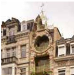
he devised has a handsome set of steps leading up to its entrance. The house has three other floors above the entrance level, each of which features large windows with curving uprights. A twisting wrought-iron plume crowns the circular loggia on the top floor, which, like the balconies on the other floors of the house, is edged with ornate railings. These were designed by Charles Van Waeyenberghe, as was the gate separating this residence from the pavement. Some observers have
